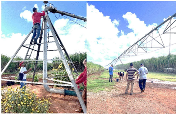
FIGURE 2. BAYATUSA-WESTERN electrical center pivot machine.
